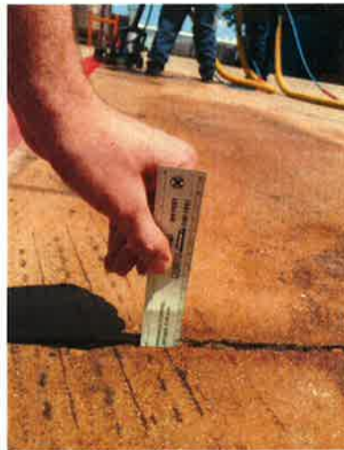
Figure 3. Removal of Impacted Material from Cement Crack with HHRU Technology
