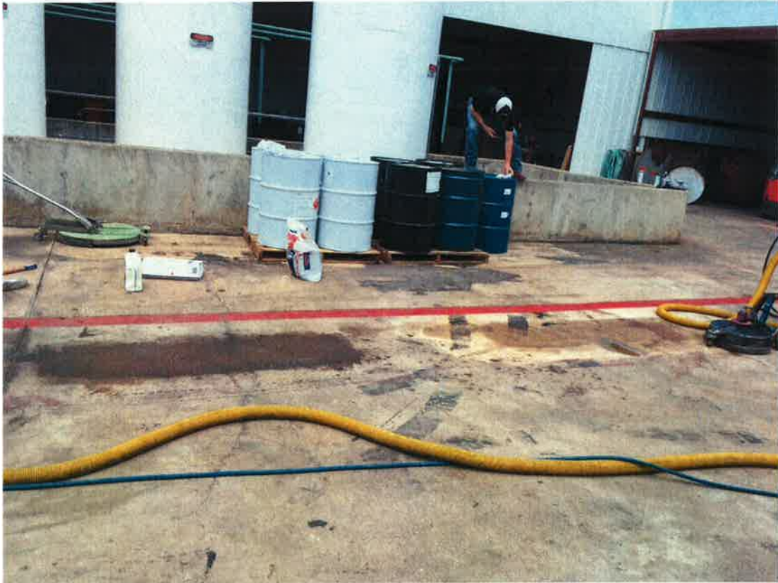
Figure 5: Paved Surface Cleaned with Absorbent/Sweep Method (on left) compared to CGs HHRU equipment (on right). (Hand held recovery unit (HHRU) is visible on the right side of the picture).
